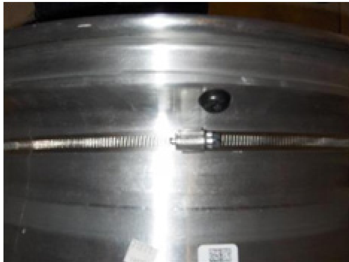
Fig. 2 - Band Installed
