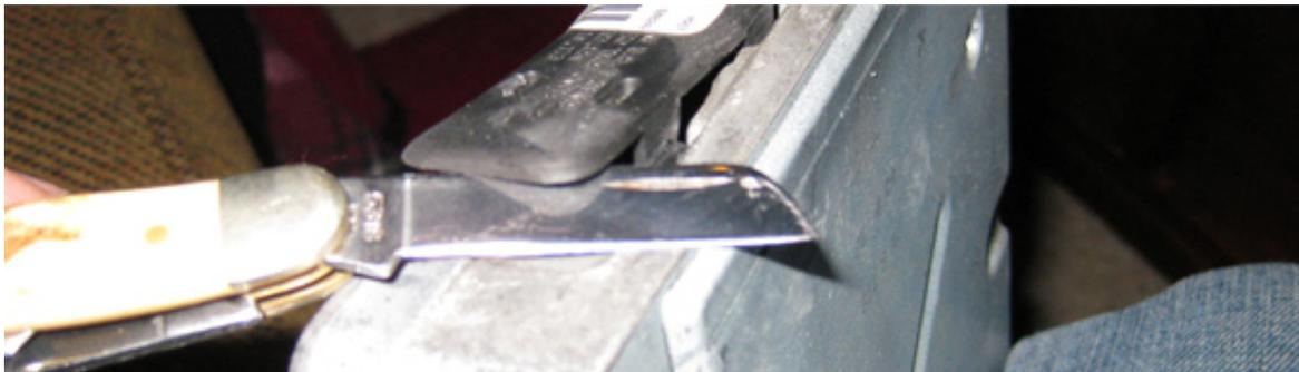
7. After that's been removed, you can clearly see that the connector is covered in some type of plastic, which needs to be removed for a proper connection.
