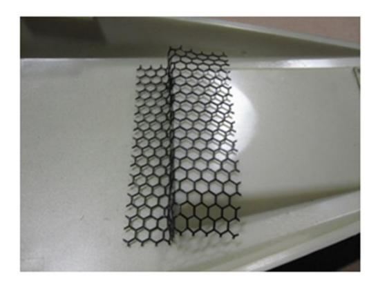
4. Remove the grille from the louver and thoroughly rub the supplied 3M Adhesion Promoter on both the surface of the louver where the grille will attach, and the grille itself. Let the Adhesion Promoter dry for a few seconds, then cut two 3" strips of tape from the 40" roll that is included and place them on the louver as shown below.
