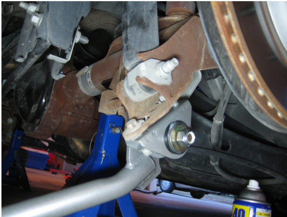
Figure 8: Axle Brackets Installed Onto Rear Axle
